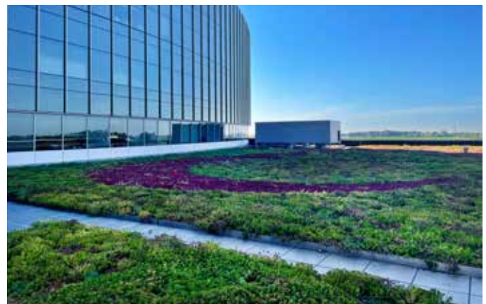
Mercyhealth Hospital - Rockford, IL
